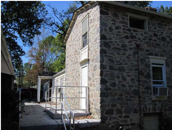
Building #1: Fieldstone building on East parcel (next to County Park). Original door below grade could indicate a previous use as a smoke house, root cellar, or ice house. Double level doors on left hand side could be another sign of large heavy items being stored in the building at some point. Bracketed eaves. Victorian style chimney could also be original.
