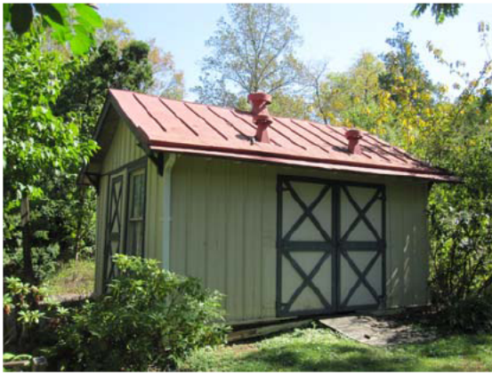
Building # 3- Original Tin roof with recessed Yankee gutter, board & batten style siding, brick foundation, Heavily bracketed soffits & eaves.
